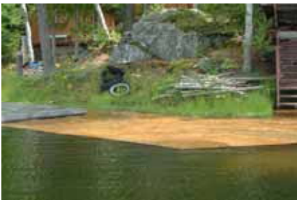
A low cement dock structure on the West Lake that was under water on July 18 th , 2004.
