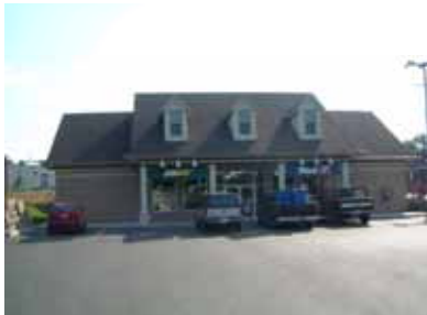
The new Mac's Milk store is a beautiful store both inside and out. The Signature Series Store is a welcome site when entering Marmora.
